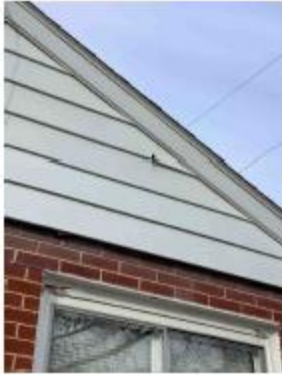
Damaged Siding
