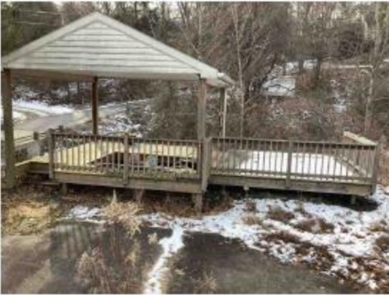
Rear Partially Covered Deck
