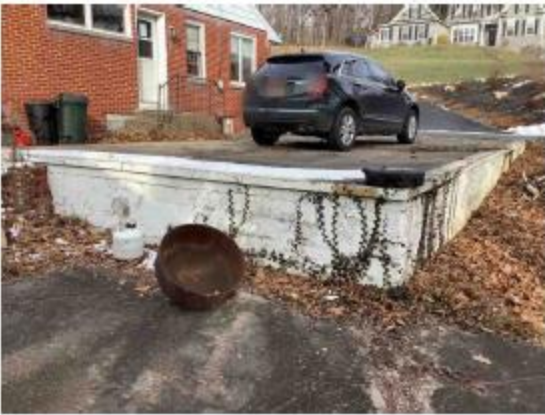
Driveway Ledge W/O Railing
