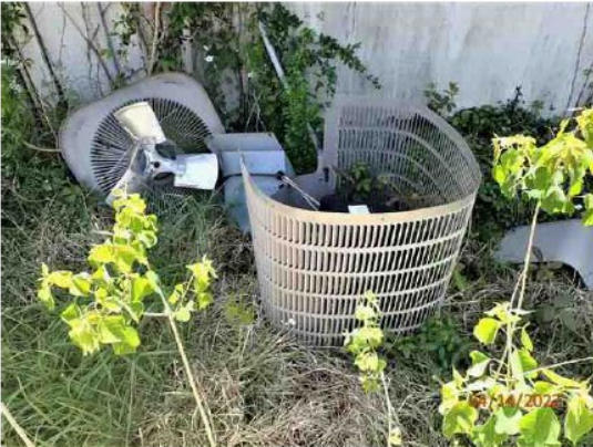
Air Conditioning Compressor
